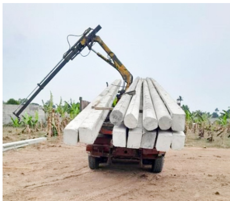
Installation of electrical poles in a host community for 33kV Power Distribution Networks.
