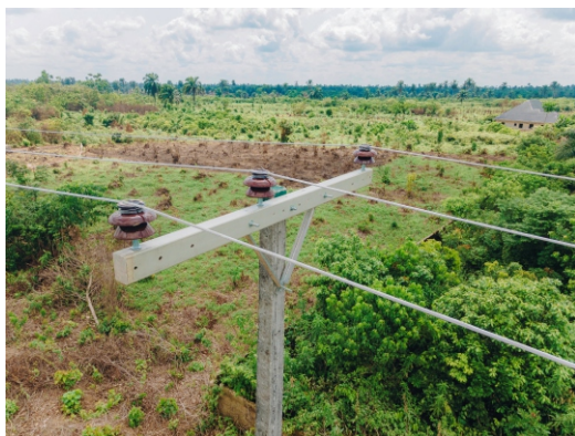
Installation of electrical poles in a host community for 33kV Power Distribution Networks.
